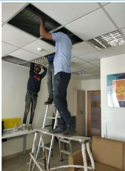
AC Unit installation in Purchase Office
