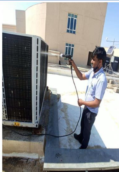
Chiller Cleaning – Right Wing
